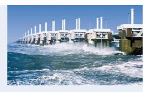
The original design was for a permanent dam to close off the 7-km-wide Oosterschelde Bay which would turn it into a fresh water lake. Environmental studies indicated that this would have a severe impact on the breeding grounds for fish in the North Sea. The dam concept evolved into a system of gates that could be raised in normal seas and lowered during storms. The gates would be supported by massive caissons buried in the seabed.
