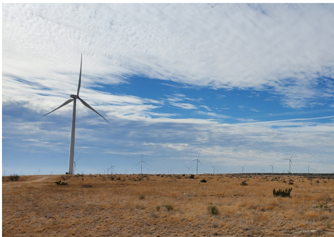
Onshore wind farm foundation monitoring
