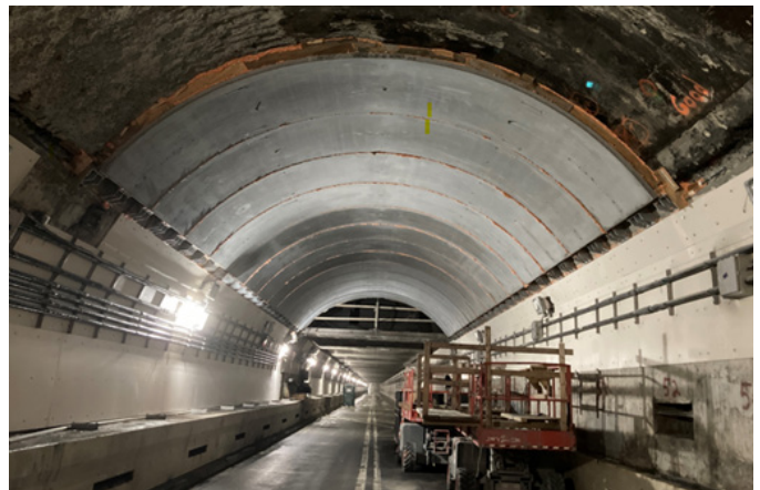
Sumner Tunnel monitoring
