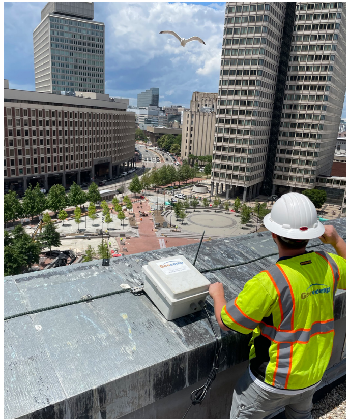
City Hall Plaza renovation monitoring
