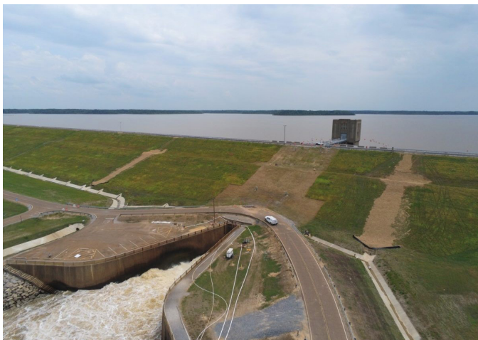
USACE Arkabutla Dam emergency repair project
