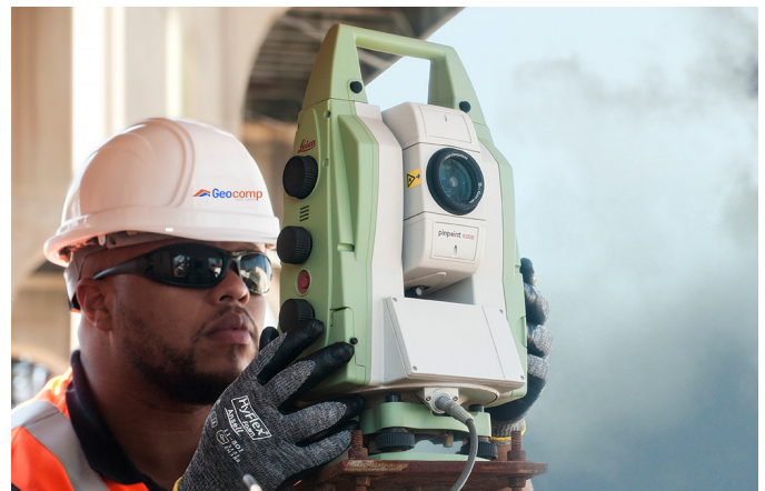
Bayonne Bridge AMTS monitoring
