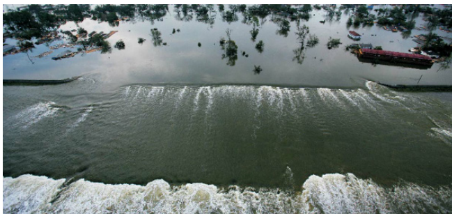
Katrina Levee failure
