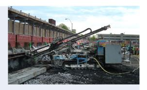
Construction for the complex began in early 2008 with the installation of deep, reinforced slurry walls to provide retaining support for a nearly 6-acre area, 48-ft-deep excavation into Boston blue clay. Excavation began in May 2008 and an extensive program of tie-back installation at 4 different depths was performed in concert as the excavation progressed. The bulk of the excavation was completed in January 2009, along with a significant portion of the 5-ft-thick reinforced concrete-base slab.
