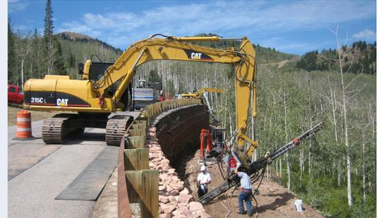
The extreme terrain conditions posed significant challenges to the on-going construction of necessary infrastructure such as roadways and utilities. The site required an extensive system of retaining walls for side hill roadway construction, vehicle bridges and ski "cross-overs". The mechanically stabilized earth (MSE) retaining walls used consisted of welded wire face elements and steel bar mats for primary reinforcement.
