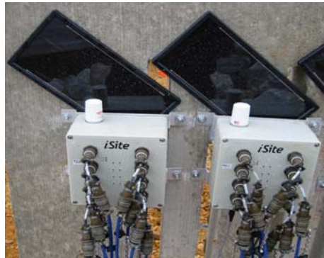
Wireless data loggers during installation
