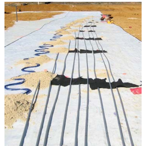
Strain gauges & rod extensometers being prepared on high strength geotextile fabric
