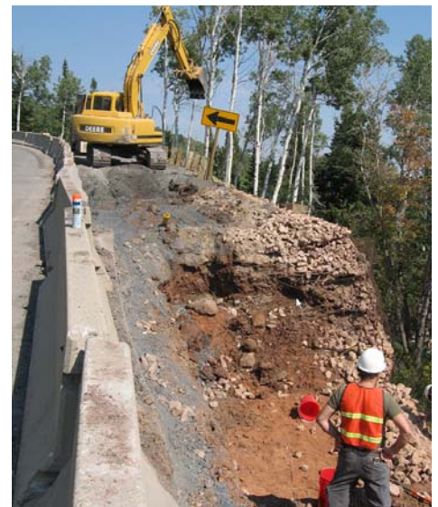
Forensic deconstruction of Hilfiker wall, 2006
