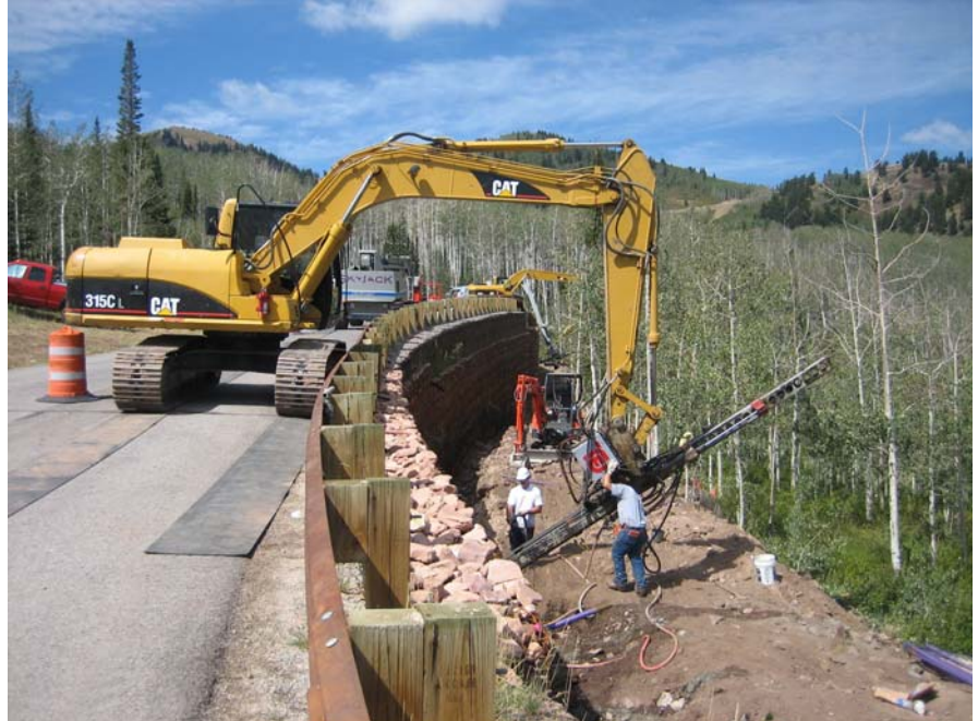
Soil nail remediation of Hilfiker wall, 2007
