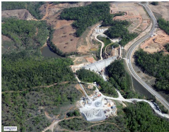
Aerial view of the dam under construction
