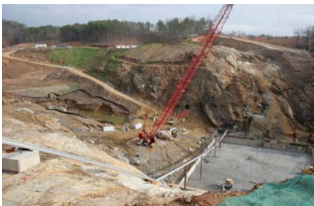
Installation of pre-cast panels and roller-compacted concrete
