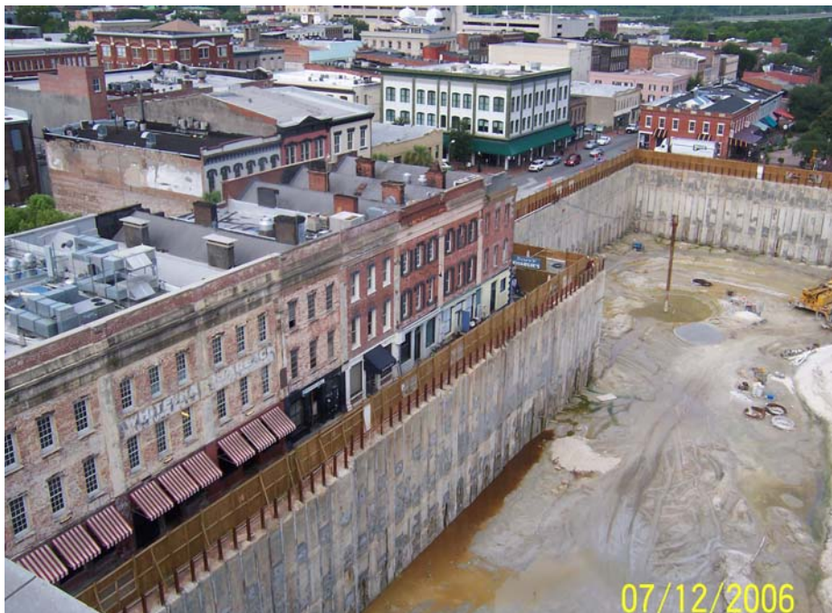
Historic buildings within feet of 45-ft. deep excavation
