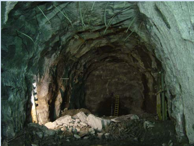
CM009 assembly chamber excavation
