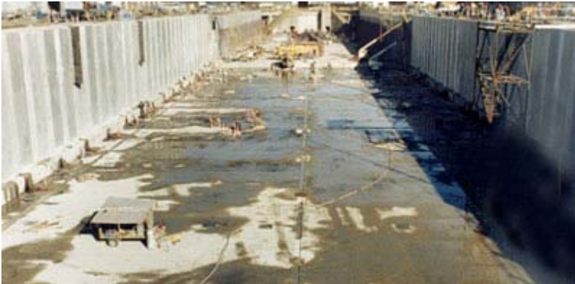
Over 1150 feet long by 180 feet wide by 60 feet deep, Dry Dock 6 is one of the Navy's largest dry docks.
