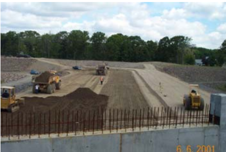
Earthwork placement and compaction
