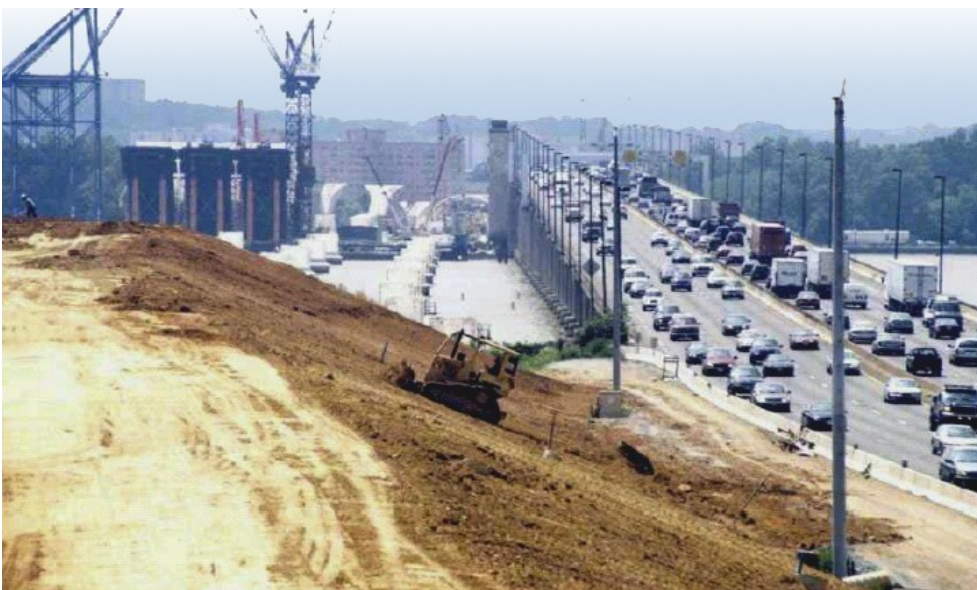
Construction work on embankment
