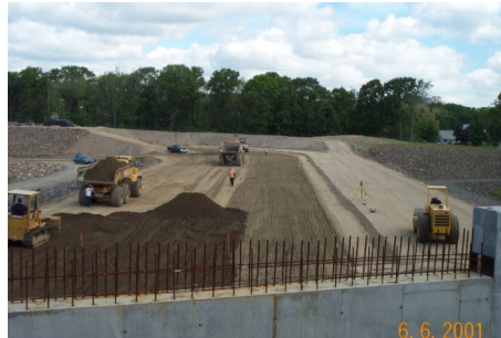
Earthwork placement and compaction
