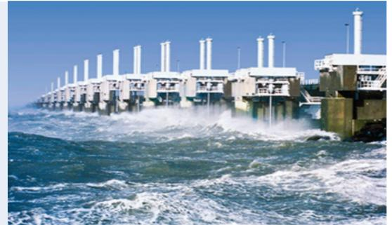
The original design was for a permanent dam to close off the 7-km-wide Oosterschelde Bay which would turn it into a fresh water lake. Environmental studies indicated that this would have a severe impact on the breeding grounds for fish in the North Sea. The dam concept evolved into a system of gates that could be raised in normal seas and lowered during storms. The gates would be supported by massive caissons buried in the seabed.
